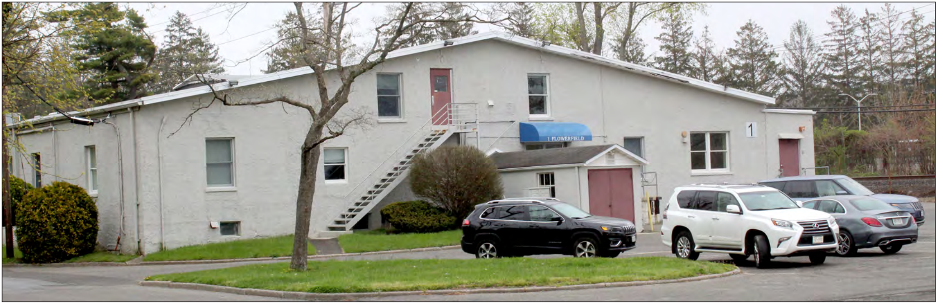
The building at Gyrodyne in St. James will not be included in the acquisition being considered by the state, which is expected to cost between $16 to $20 million.
